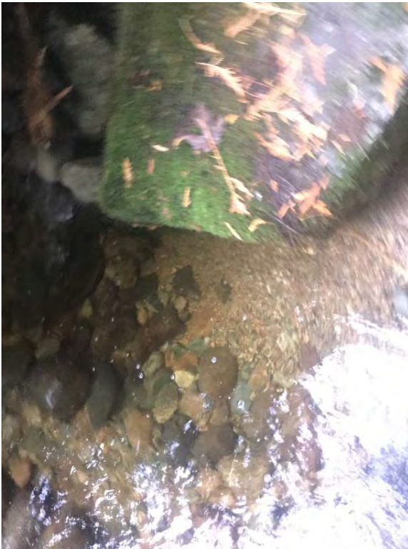
Right Bank Abutment when facing downstream
