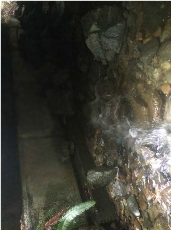
Right Bank Abutment when facing downstream
